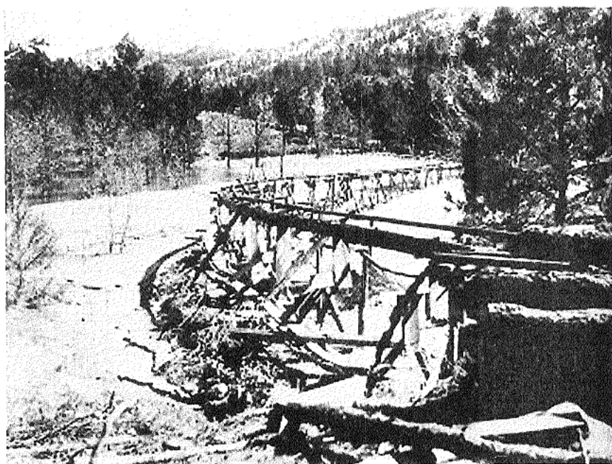
Eight inch wooden pipe followed Rich Gulch to the filter plant
