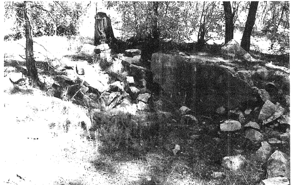
The ice house was built by Alfred Curtis and his son Fred. When it got cold enough they cut ice from the creek. Otherwise, they would compact snow.
